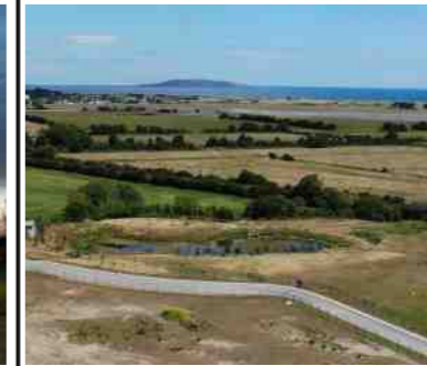
Attenuation pond and Wetland Park under construction
