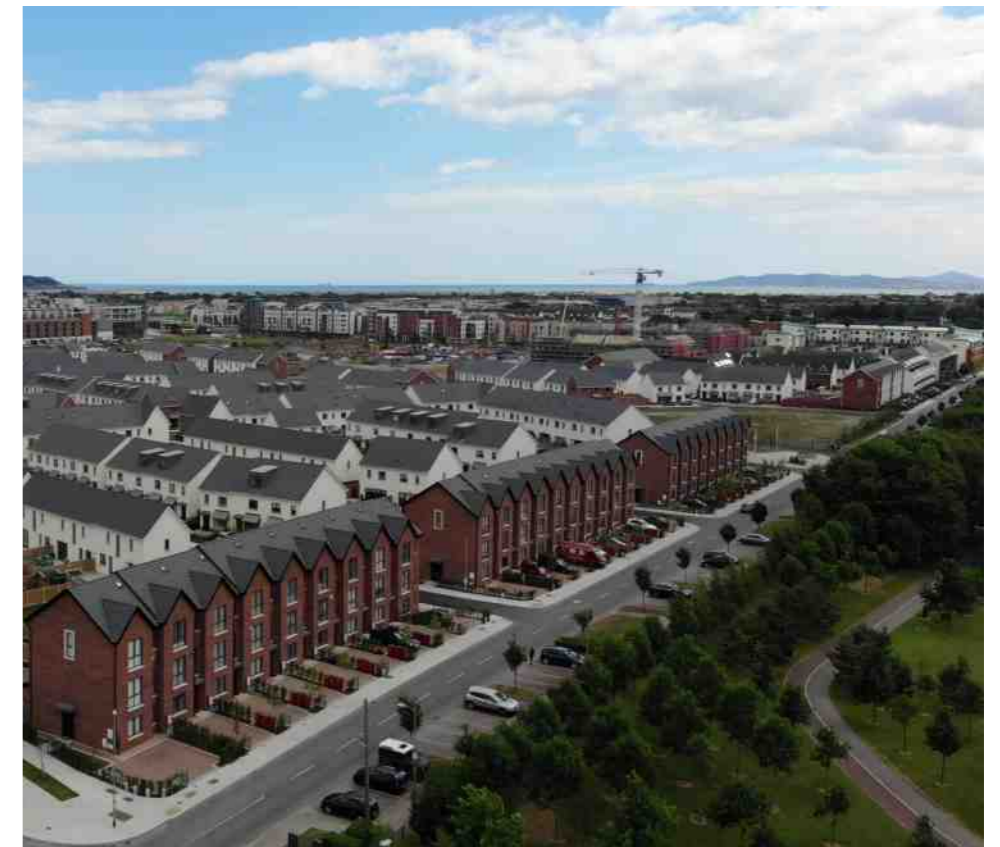
Medium density single family houses along Park Avenue
