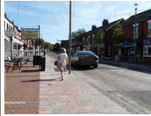
Flush surfaces encourage driver caution
